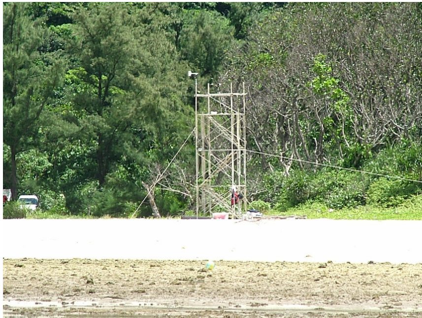
Photo 2. Installation set-up of anemometer
