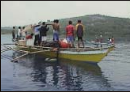
Installation of marker bouys, Bantayan
