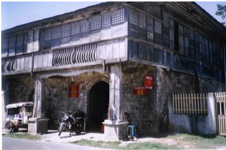
Figure 14. An eighteenth century house in Dumanjug, western Cebu showing “capis” shells used for window construction. The first storey of the building was constructed out of coral stones.
