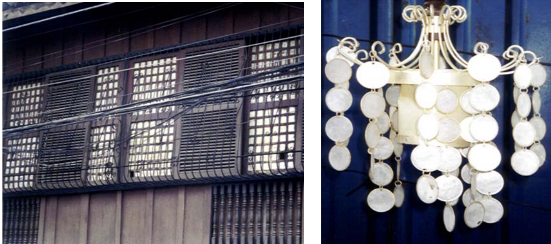
Figure 13. Ancestral house Casa Gorordo Museum (Left), built from “capis” shell Placuna placenta . Right photo shows the wind chime made from similar material.
