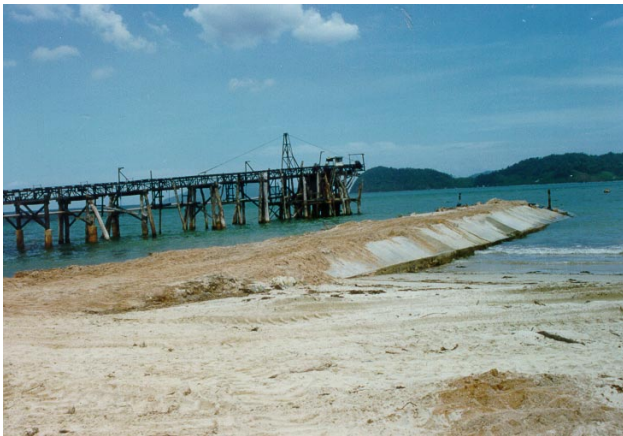
DOWNSIDE OF DEVELOPMENT. Mining for silica and the construction of a pier have caused siltation and beach erosion in sitio Sta. Cruz, Barangay Caruray.
