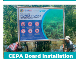
CEPA Board Installation
