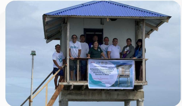
31 January 2025 – CCEF formally turned over the newly renovated MPA Guard House of the Hingotanan West Fisherfolk Association (HIWeFA) in Bien Unido, Bohol. With support from Booth and Partners, the MLGU, and BLGU, the project benefits 30 fisherfolk members by strengthening their capacity to protect marine resources.
